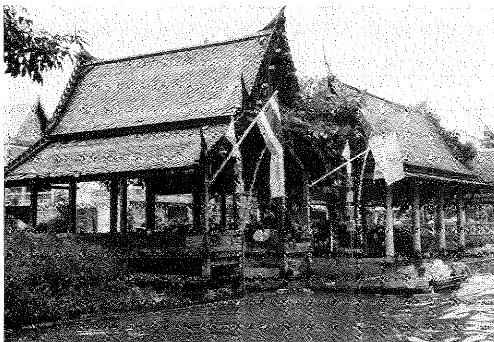
Architecture of central Thailand, the region in which Nongyanang is located
